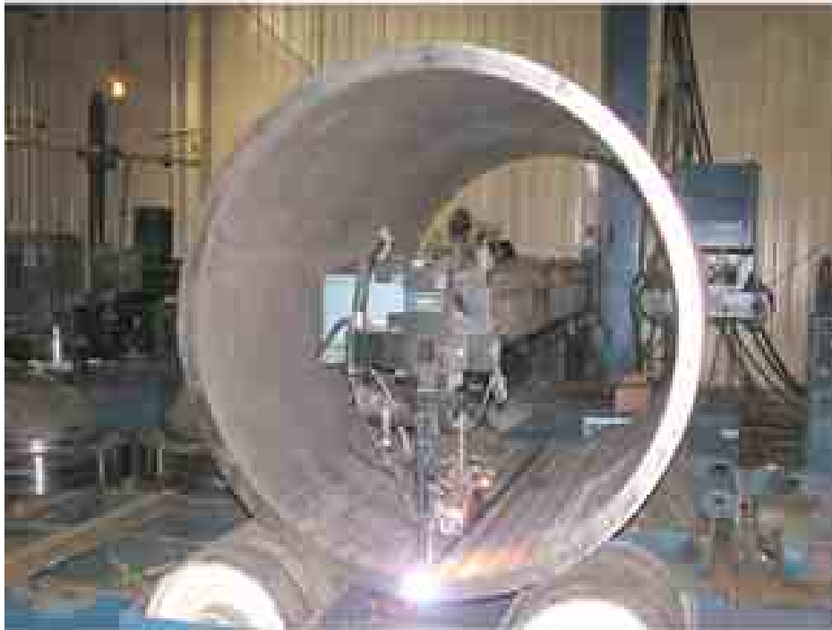
Longitudinal seam welding on the 316 stainless steel inner vessel
