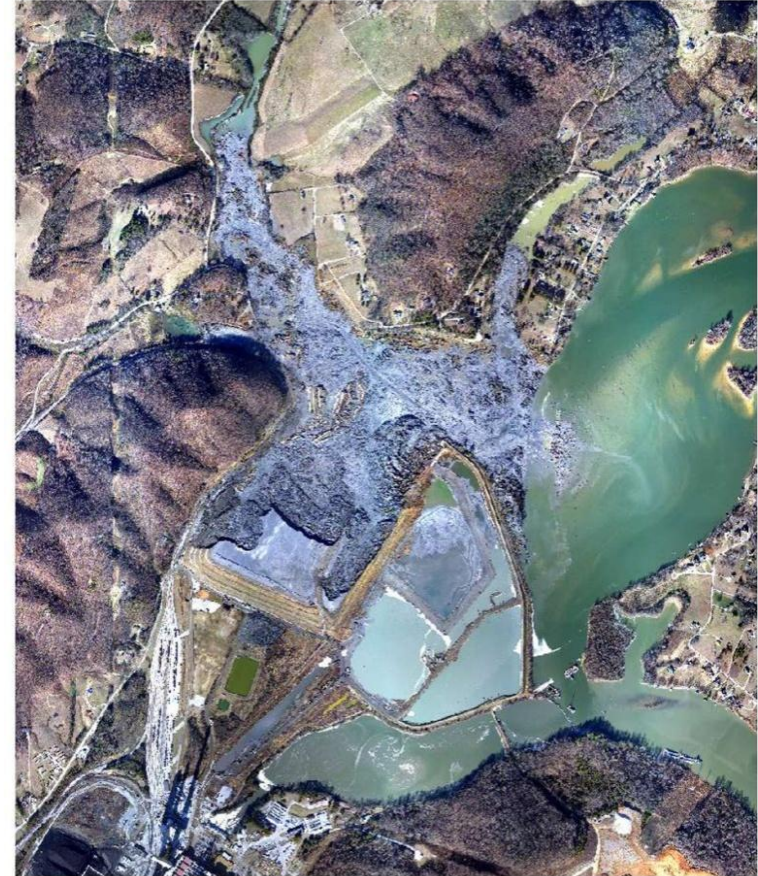
Aerial Image of Kingston Ash Slide 12/30/2008
