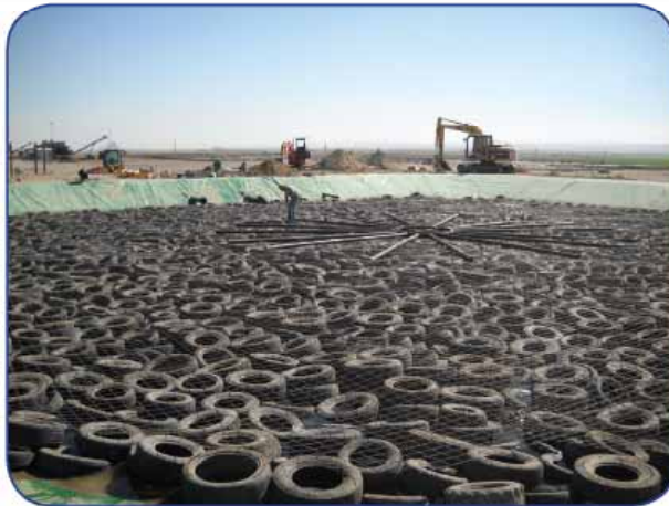
Photo taken during construction - 2009
