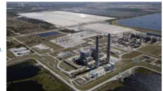
FPL Hybrid Solar Thermal and Gas Turbine Power Plant
