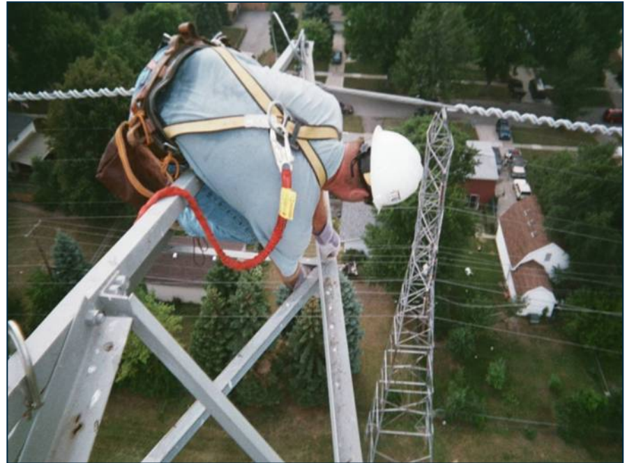
Physical Inspections 1,441 towers inspected vs. prior 5-year annual average of 952
